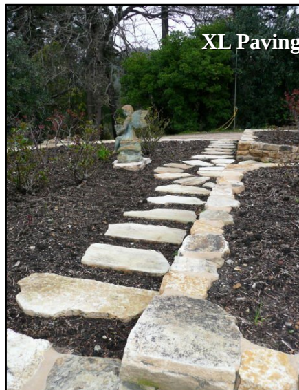
Paving cut by mason to create tighter mortar joints
