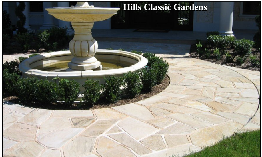
Paving cut by mason to create tighter mortar joints
