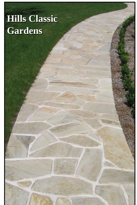
Paving cut by mason to create tighter mortar joints
